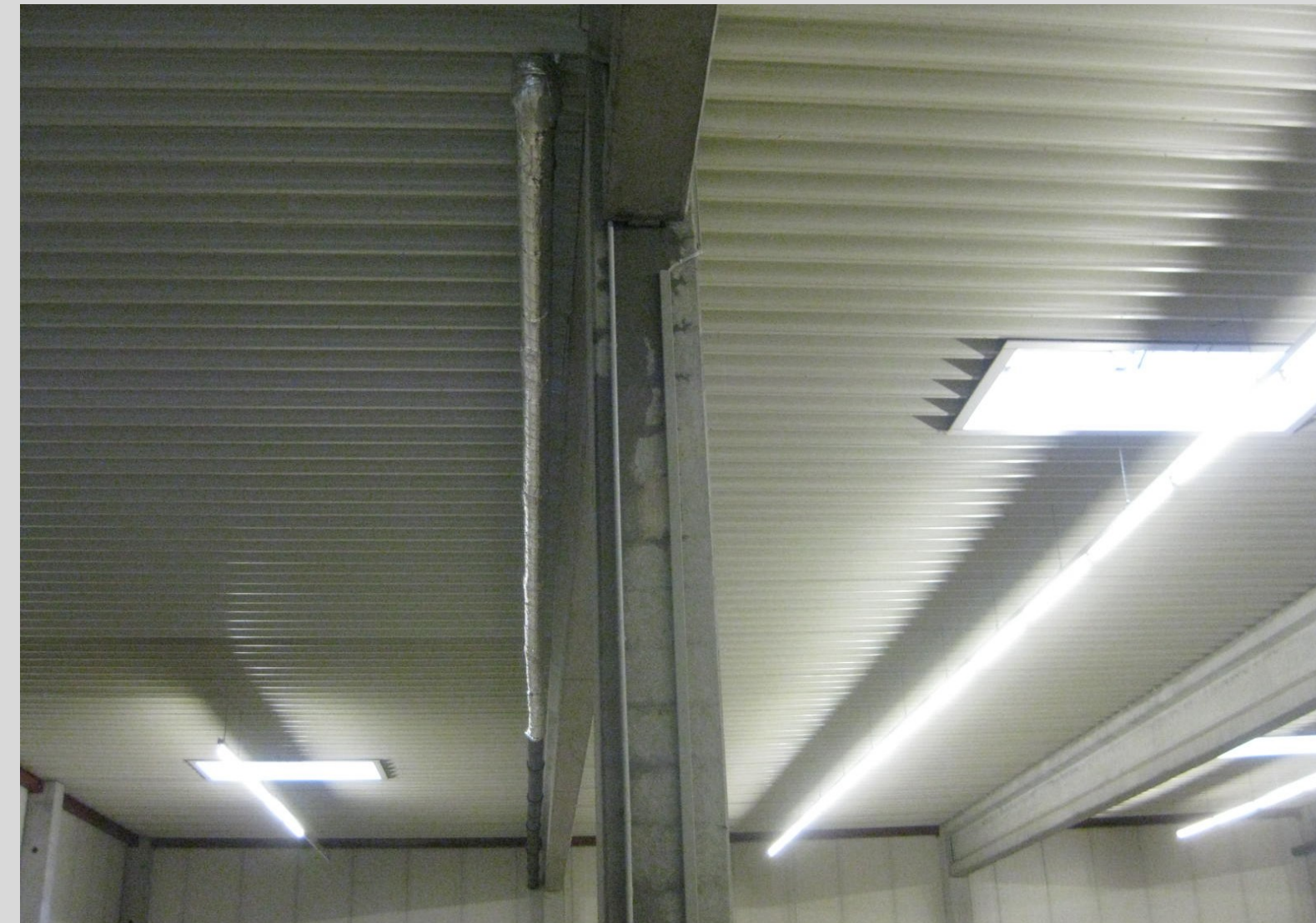
Photo 2: Horizontal PVC-downpipes
