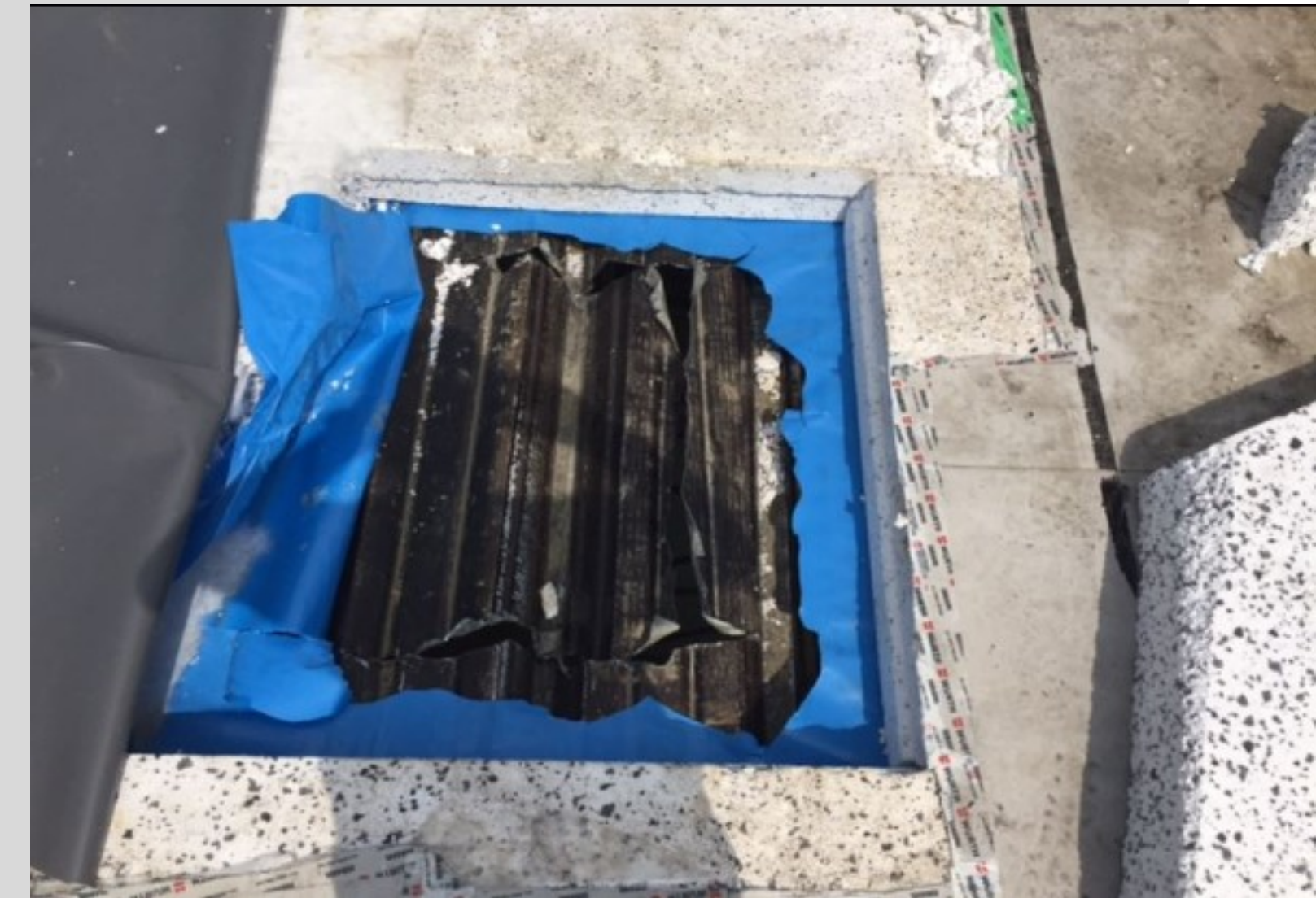
Photo 3: Ongoing repair at the time of survey
