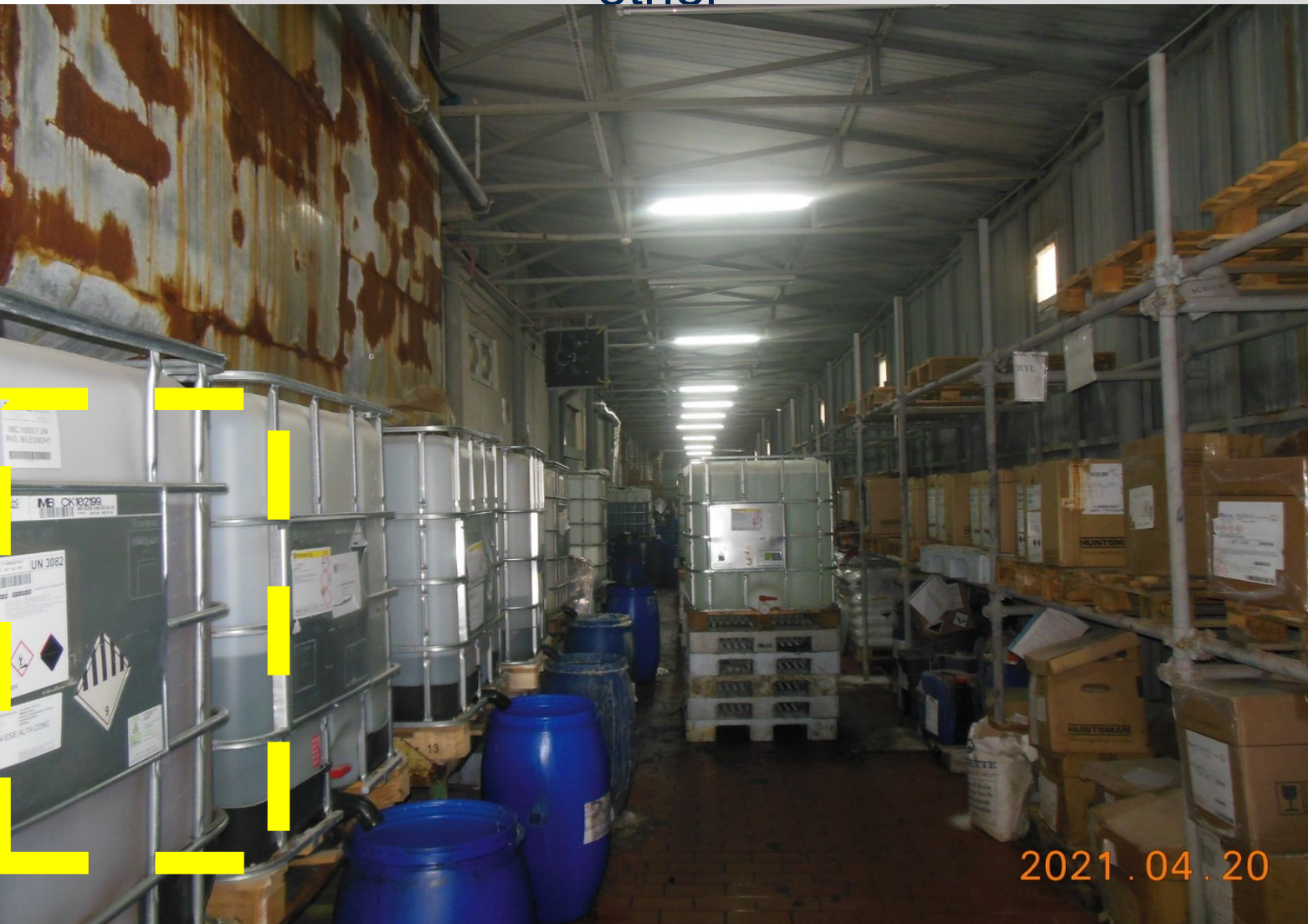
Photo 1: Different fire loads (cardboard, hazardous goods) directly next to each other
