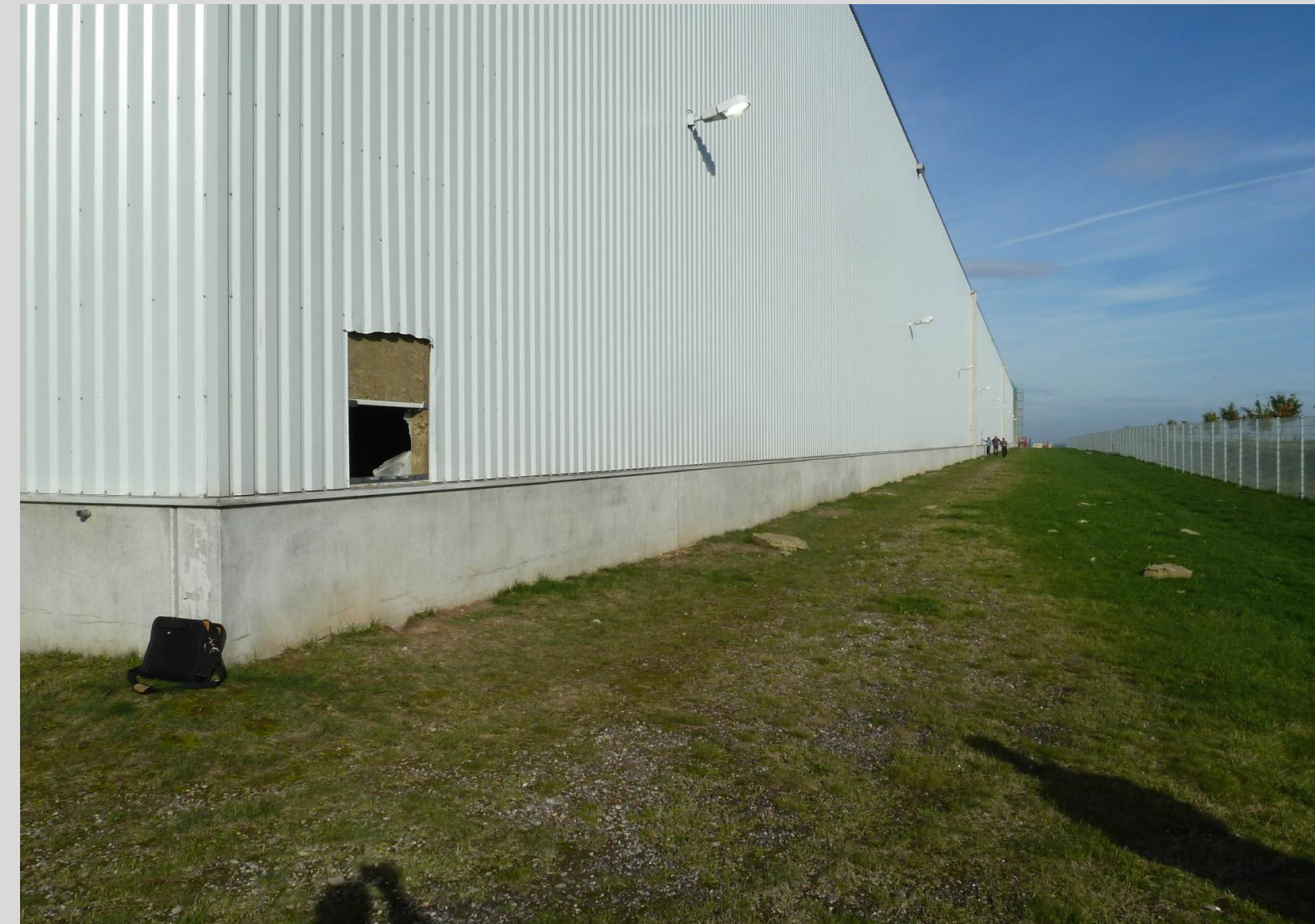
Photo 2: Closer view of outer wall
