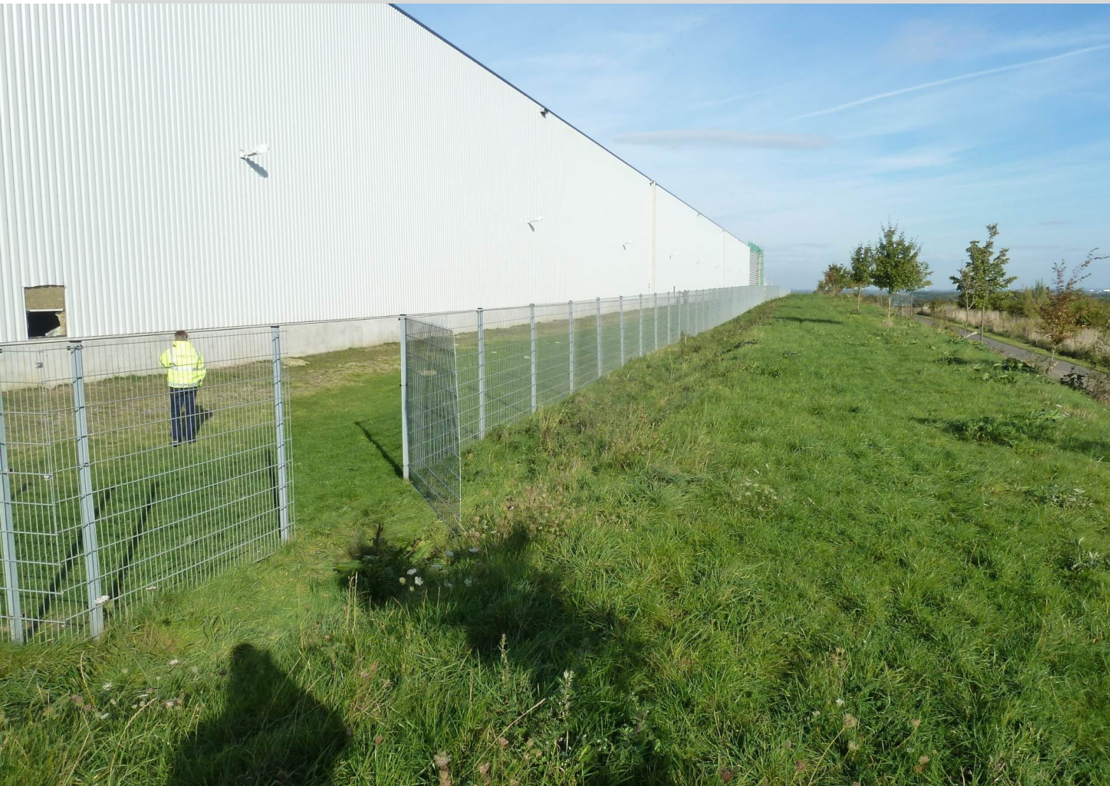
Photo 1: Fence and outer wall opened
