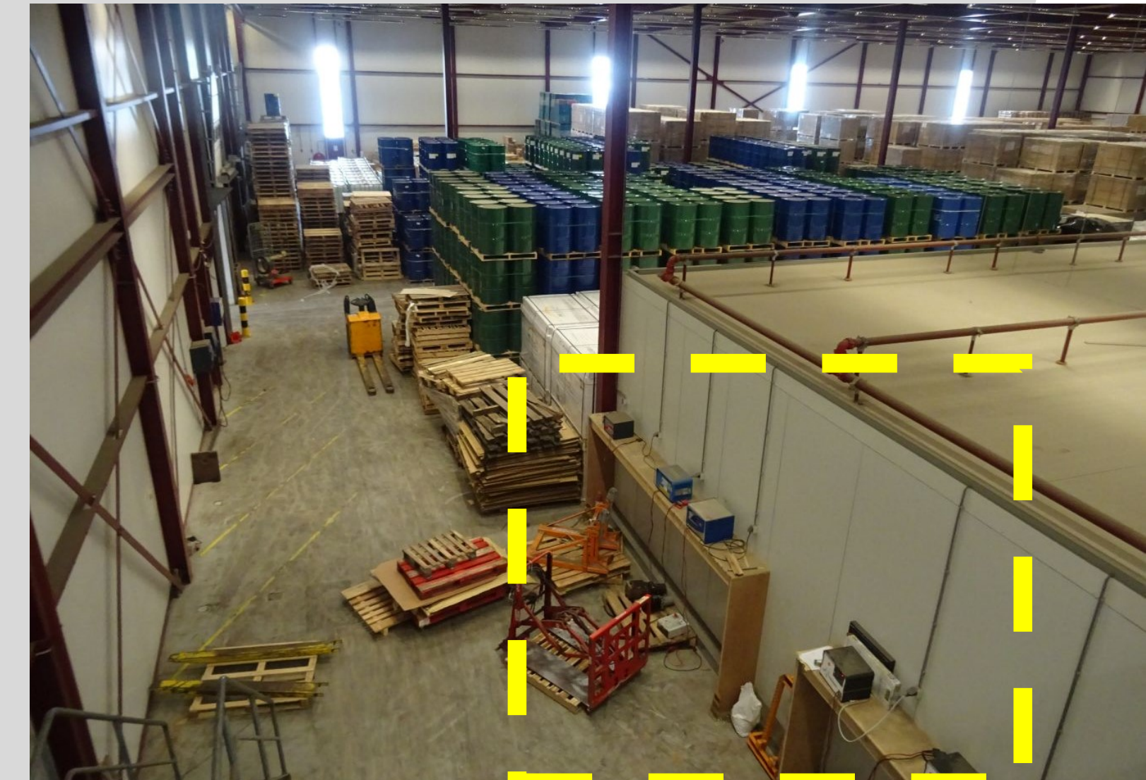
Photo 3: Ignition sources next to avoidable fire loads
