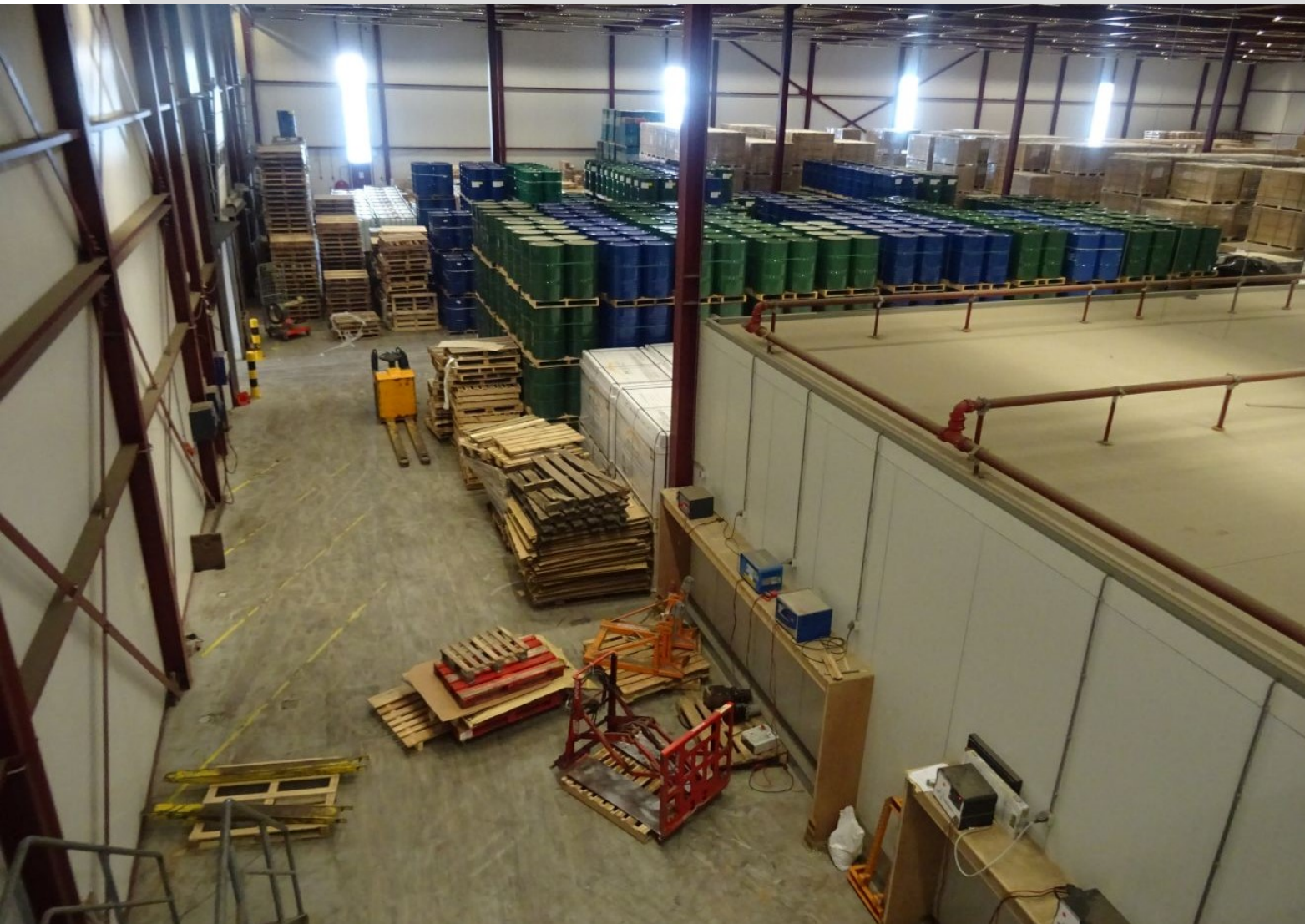
Photo 1: Fire loads and charging stations
