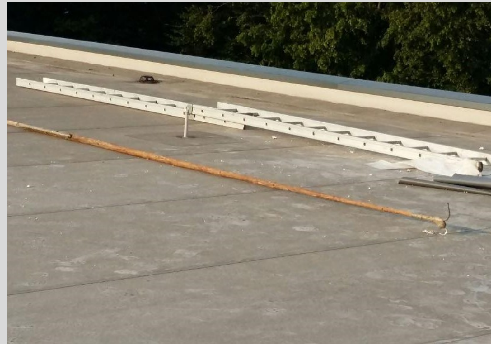
Photo 2: Ladder and Tools were left behind
