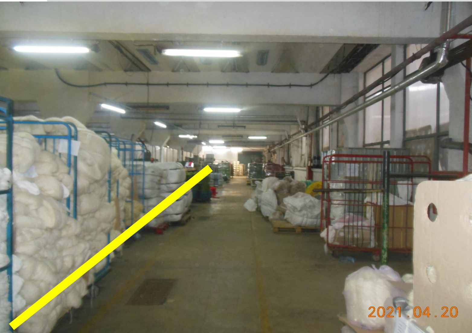
Photo 1: Fire loads in a long row
