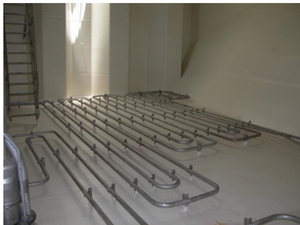
Epoxy coated cargo tank
