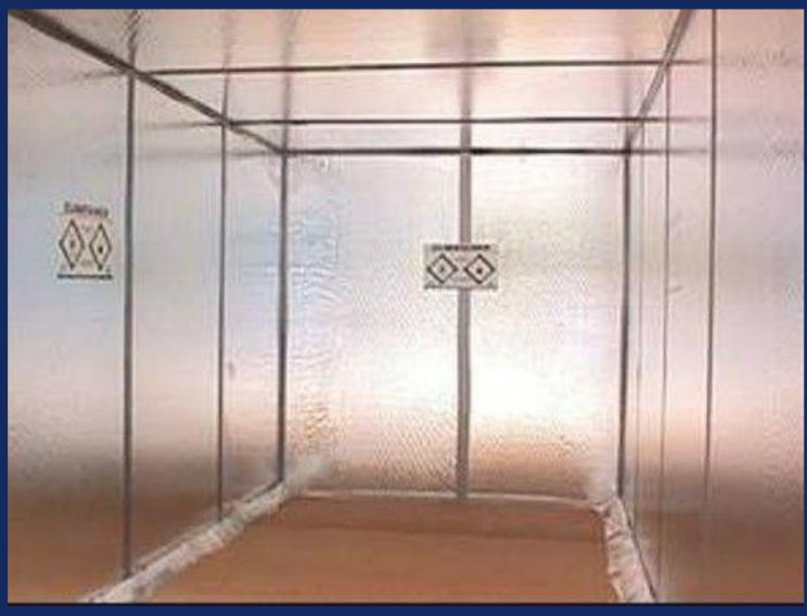
Adding an insulation wall in dry containers
