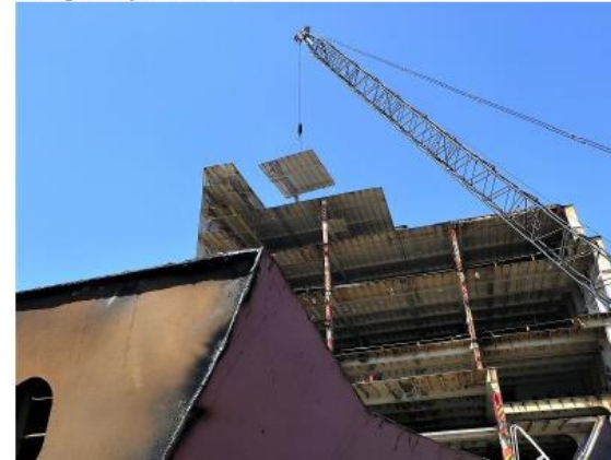
Lifting deck plates to shore
