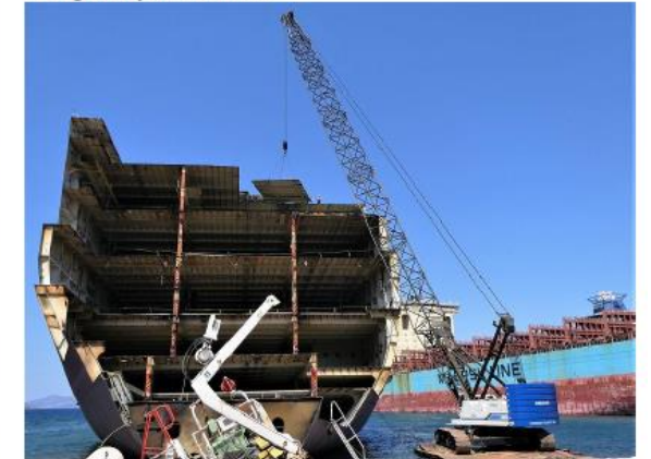
Lifting deck plates to shore
