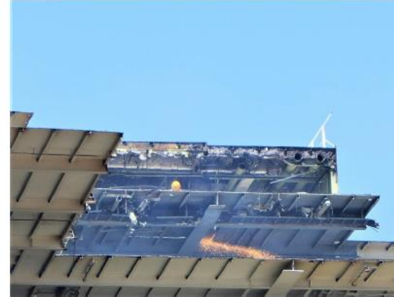
Cutting main deck
