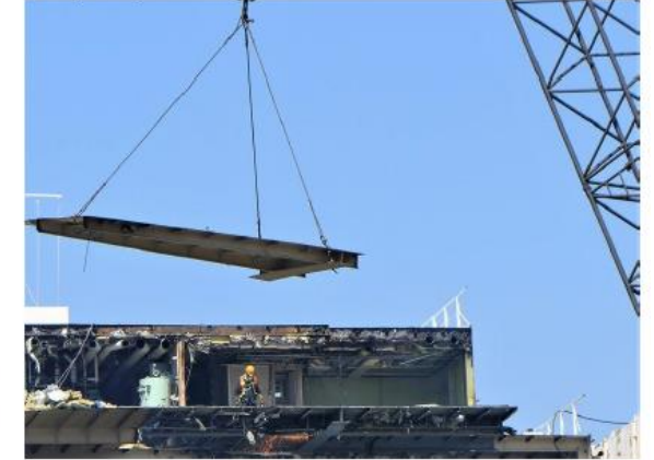
Lifting deck plates to shore
